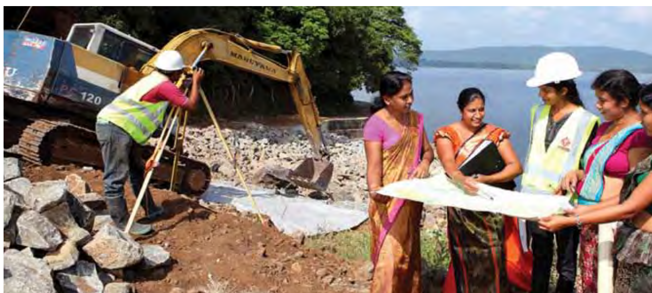
Dam under construction in Sri Lanka. ©Lakshman Nadaraja/World Bank
