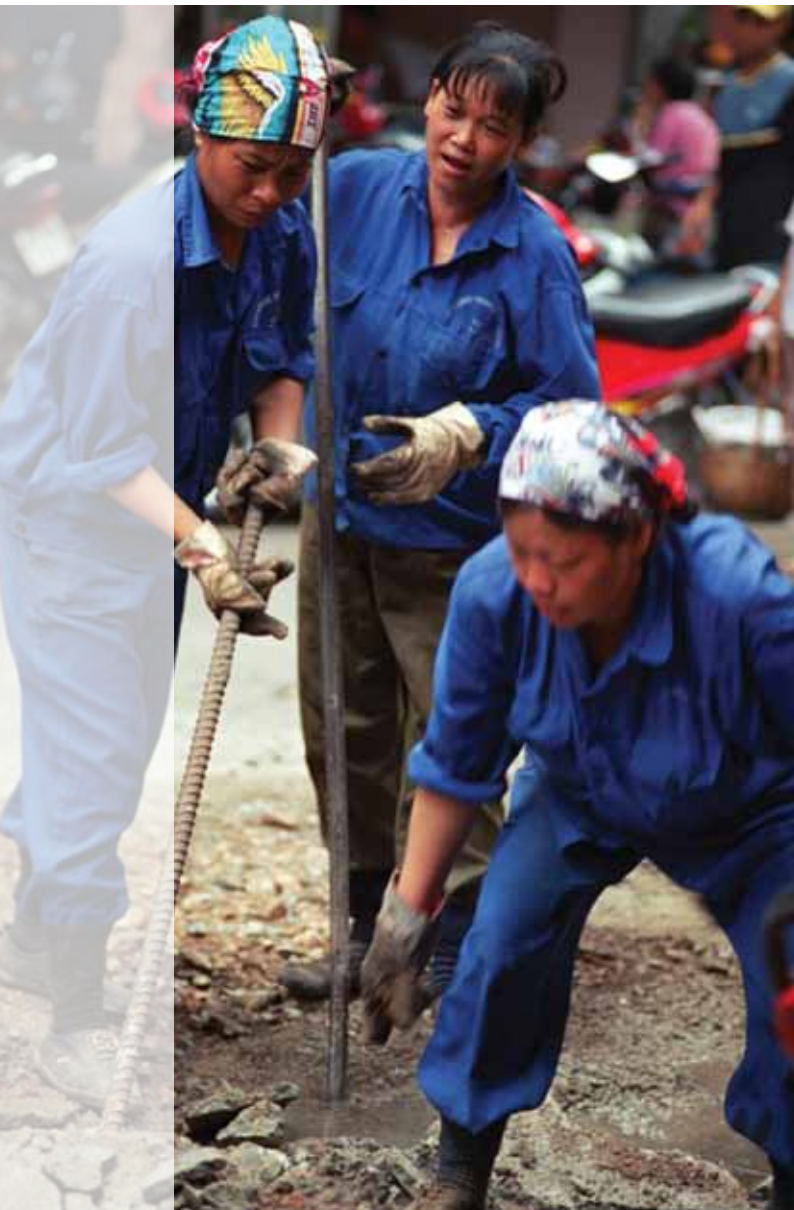
Women repairing a road in Hanoi. ©Tran Thi Hoa/World Bank
